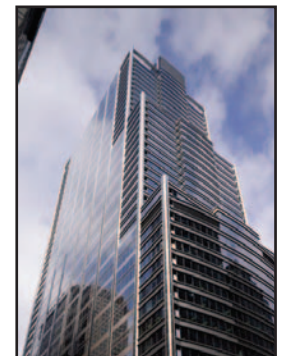
Extruded aluminum components for the tower’s curtainwall were custom-designed in partnership between design engineers, extruders, and die makers.
