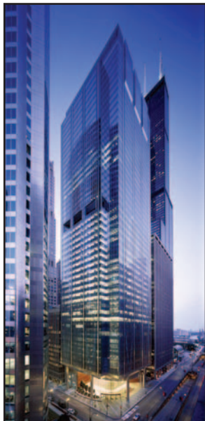
The 111 S. Wacker building incorporates aluminum extrusions into every aspect of its green design.
